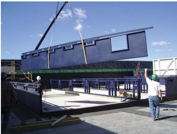
Special Height RSC to allow duct to pass horizontally through the curb.
