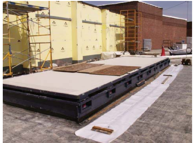
RSC with optional Acoustical Package installed prior to rigging unit
